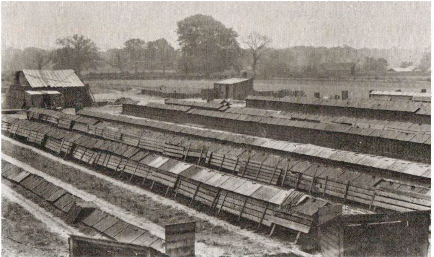
Butterfield's brick-works, Caddington – drying bricks under cover before firing
